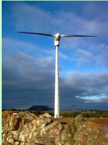
Figure 22, 275kW Vergnet wind turbine (East Lothian, Scotland, panoramio.com)
