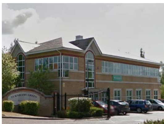
Turnhams Green offices
